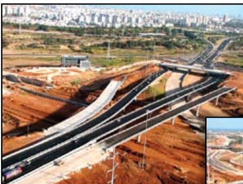
Ein Hakore Interchange with traffic on mainline structures. Courtesy of Sivan Aerial Photo.
